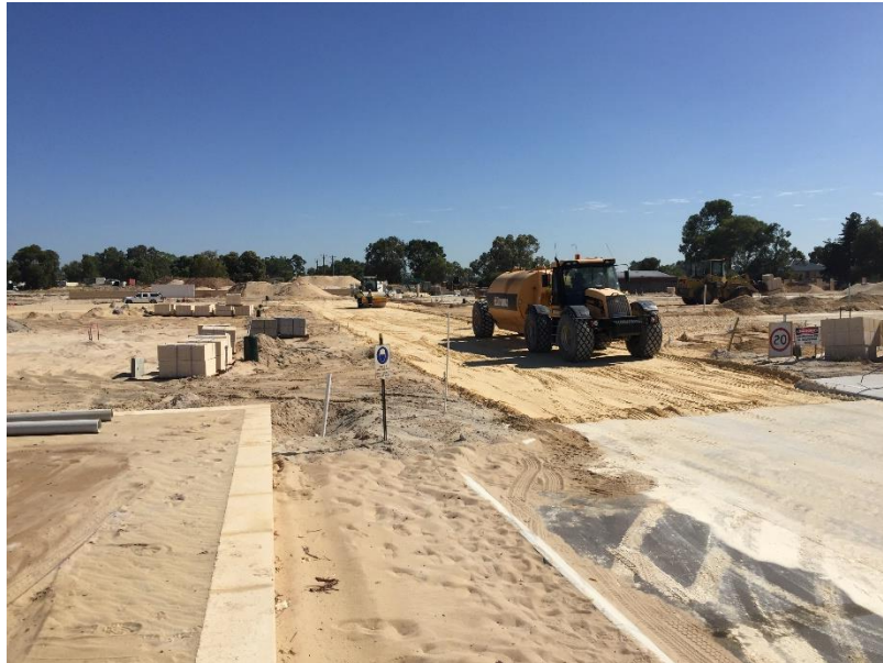
Lots under construction in stage 1P.
