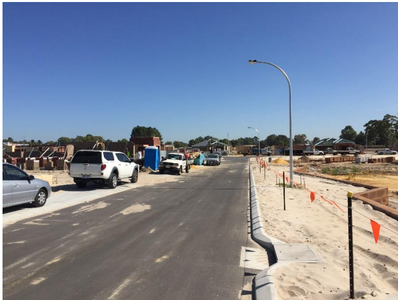
Stage 10 display village under construction.
