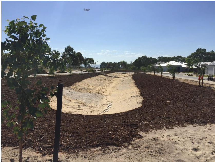
Landscaping works under construction on Cranleigh Street.
