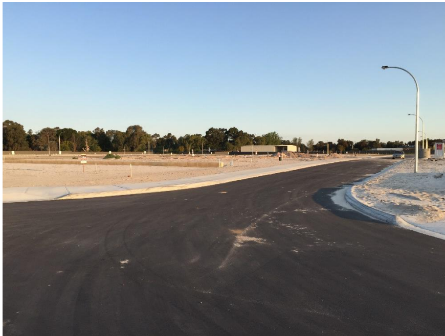
Completed lots in stage 1S.
